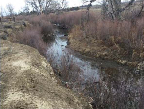
Photo 13. Looking northeast at stream S-1n in the southern portion of the project study area. Note the large amount of stream bank erosion and slumping occurring on the stream bank along the western bank (left).
